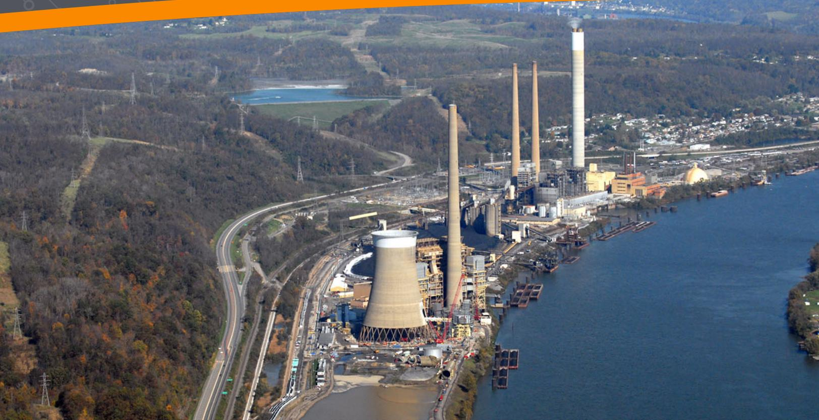
Coal arrives at the station by truck, rail, or barge and is stored in the coal yard. Conveyor belts carry the coal into the plant, where pulverizers grind it into a fine, talcum-powder-like consistency. The powdered coal is injected into the steam generators, where it burns at high temperatures, turning water into steam.
