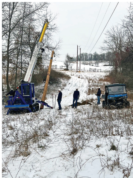
Firelands Electric crews use the cooperative's tracked digger to help set a new utility pole near State Route 603 in Richland County.
