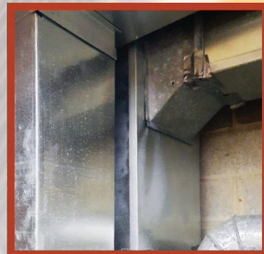
Never use duct tape to seal air leaks. It isn't made to stand up to the extreme temperature changes of an HVAC system and won't last. Always use mastic, foil tape, or other products specifically made for ductwork.
