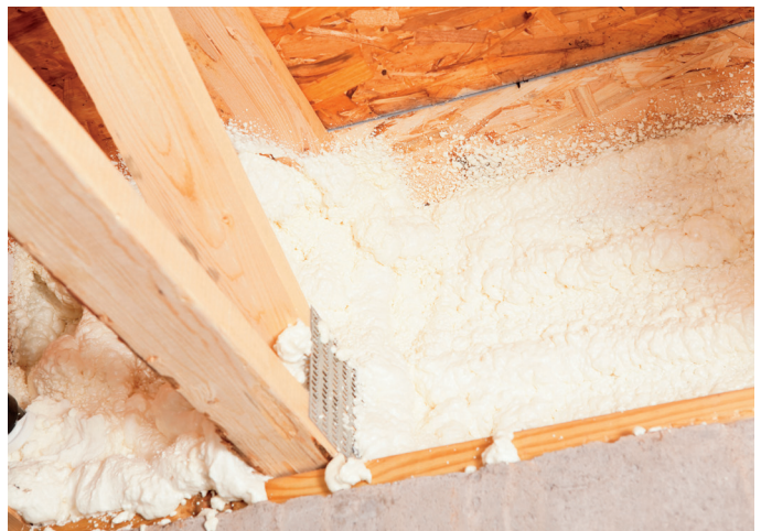
Box sills, the area between the main floor and the basement wall, can be the site of significant energy loss if they're not properly insulated.
