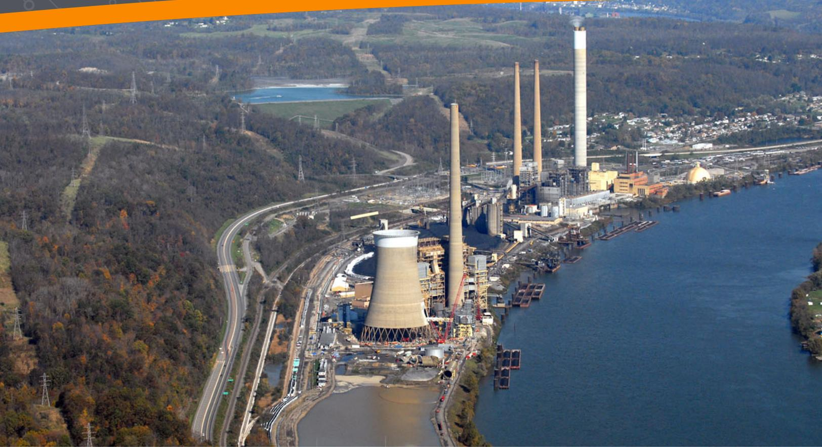
Coal arrives at the station by truck, rail, or barge and is stored in the coal yard. Conveyor belts carry the coal into the plant, where pulverizers grind it into a fine, talcum-powder-like consistency. The powdered coal is injected into the steam generators, where it burns at high temperatures, turning water into steam.
