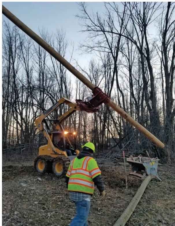
A Firelands Electric Cooperative crew installs a new pole during part of the rebuild work over the past year.
