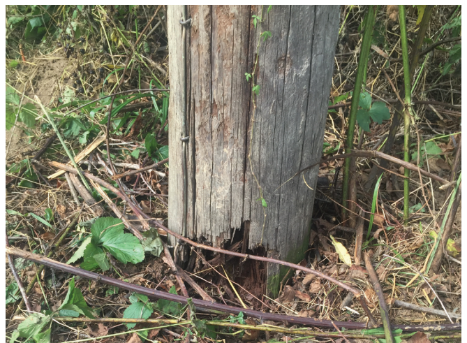
Periodic testing helps Firelands Electric Cooperative identify utility poles that are weak or damaged, like the one shown above. The co-op adds these poles to its work plan so that they can be replaced.
